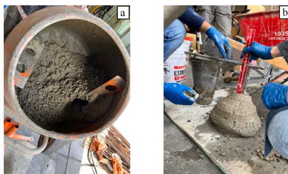
Fig. 10. Concrete mixing (a) and slump measurement (b).
