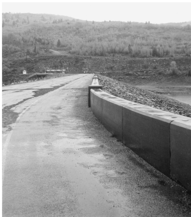
FIG. 1. Overall View of Wall Panels (Facing South)
