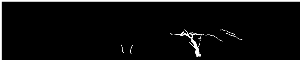
Figure 23. Image processing for cracks in BDRA beams.
