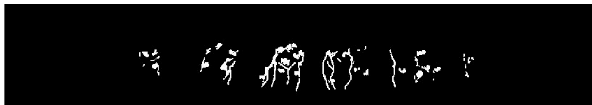
Figure 10. Image processing for cracks in SBDCM (10-3) beams.
