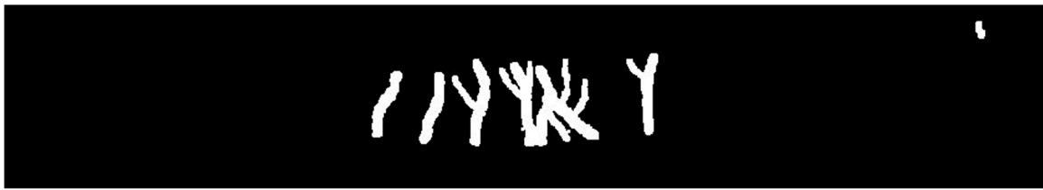
Figure 12. Image processing for cracks in BDCM (15-1) beams.
