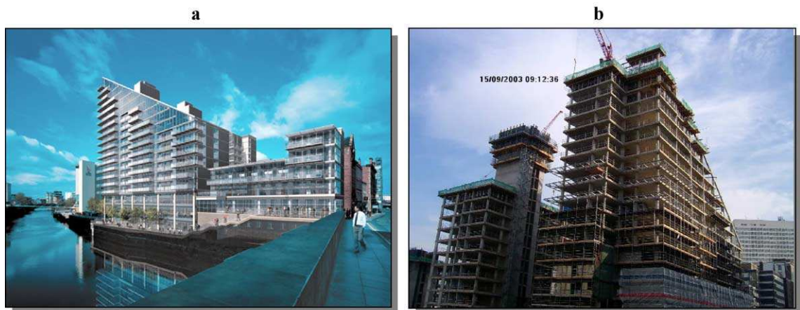
Fig. 13. The online case study. (a) 3D view, (b) project under construction.
