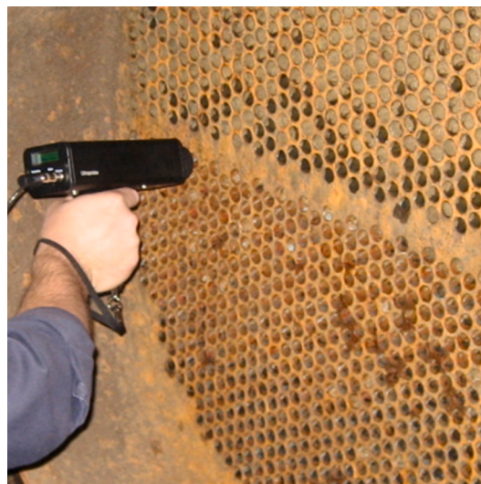
Fig. 21. Ultrasound leak detection at the tube-to-tubesheet joint [309].
