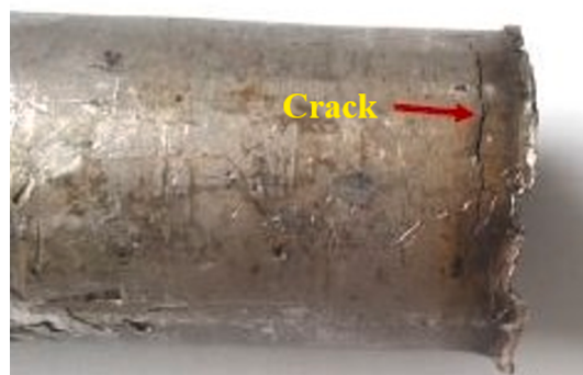
Fig. 2. Crack in the outer tube surface close to tube-to-tubesheet joints [12].
